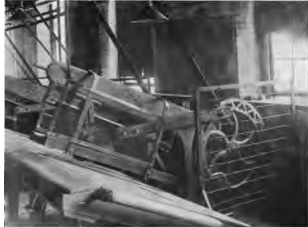
Fig. 2. Guards for Glazing Jack.*
